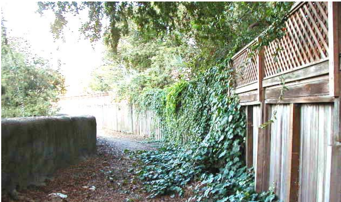
Photo 2-4-- Floodwall Demolition and Reconstruction. Photo is looking downstream, at the Palo Alto top of bank. The existing floodwall is at photo left, with existing property fences at photo right.
