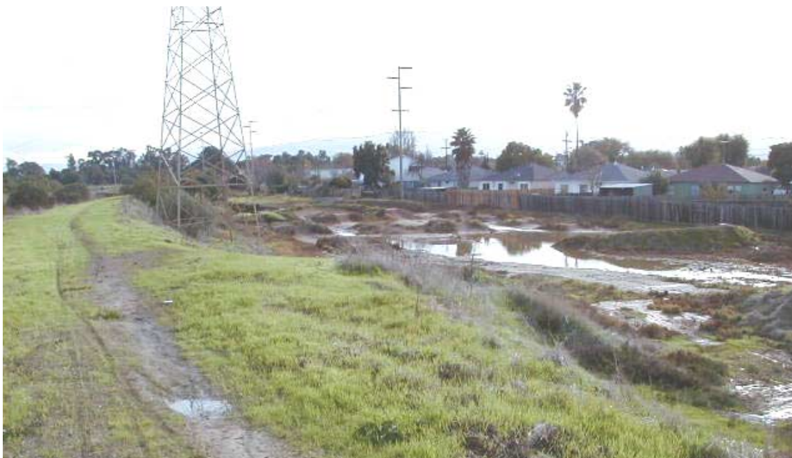
Photo 2-1-- Levee Restoration portion of the project, with the northern levee (San Mateo County) at photo left. The closest residences in East Palo Alto are to the right of this levee. This levee is made of compacted earth, and the maintenance road on top of the levee is unpaved.
