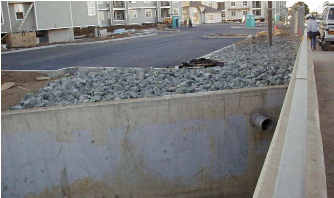
Photo 2-5-- Floodwall Demolition and Reconstruction. Photo is looking from the West Bayshore Bridge, looking at the East Palo Alto side of the creek and the CALTRANS wier.
