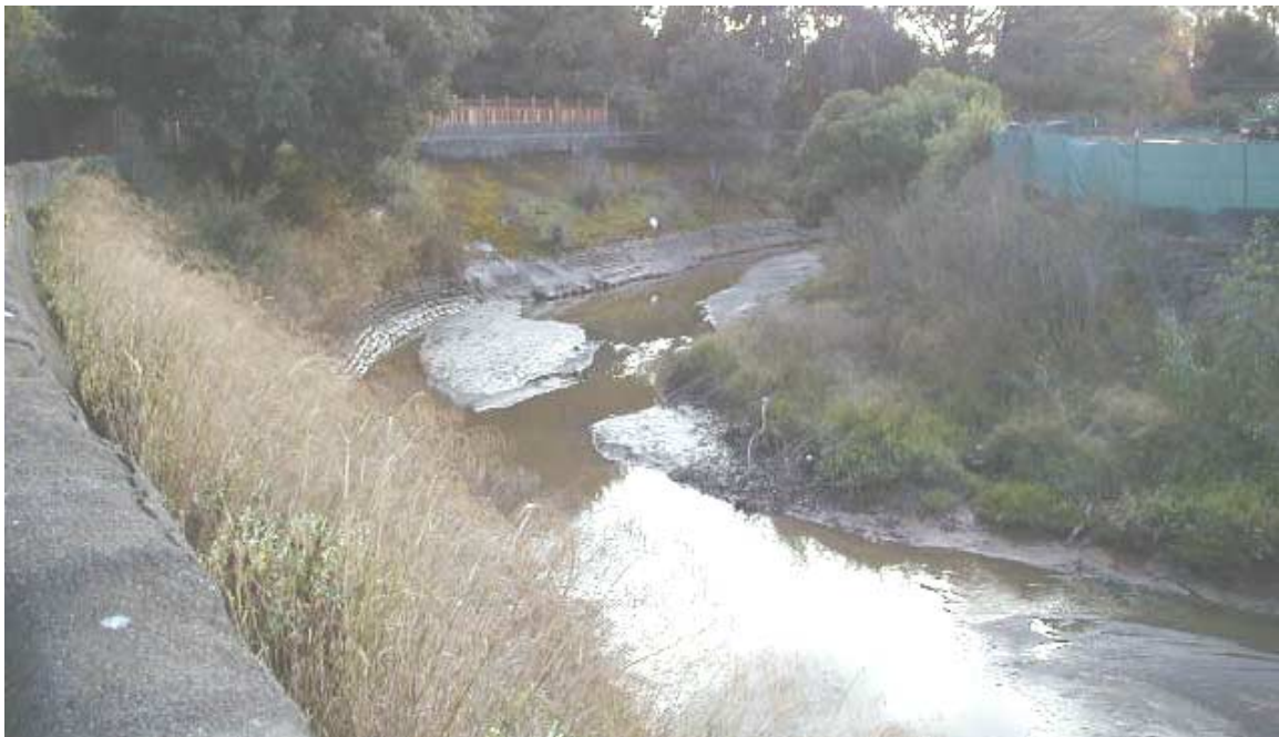
Photo 2-6-- Floodwall Demolition and Reconstruction. Photo is looking upstream, at the Palo Alto top of bank. The existing floodwall is at photo left.
