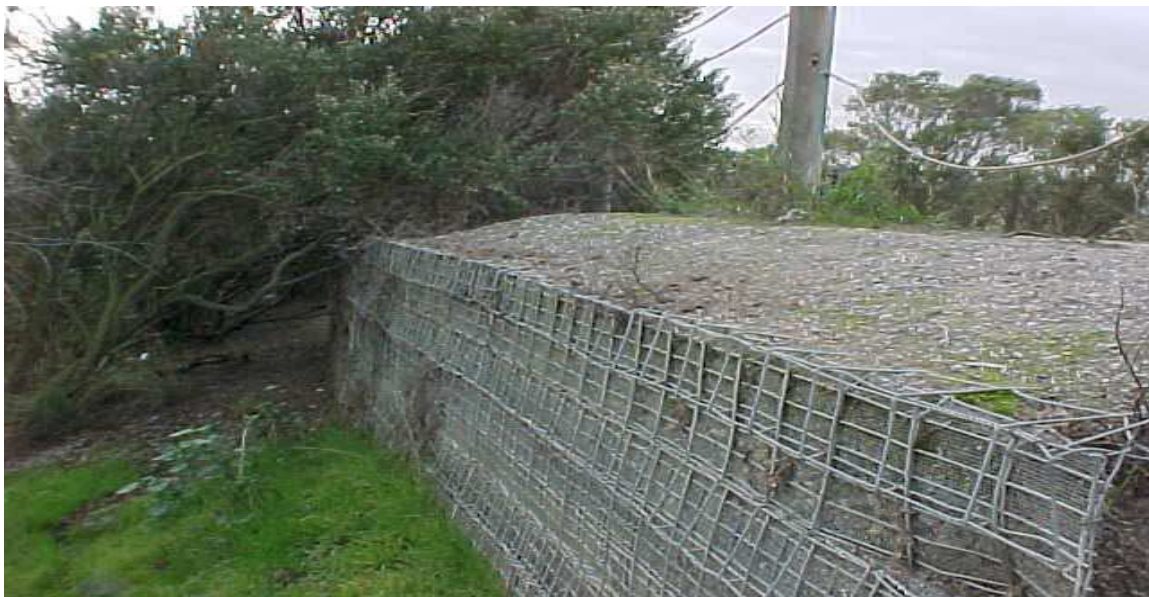
Photo 2-7-- Photo of Hilfiker method, on another project. The Levee Reconstruction project is proposed to use this method adjacent to all sensitive biological areas as to not increase the toe of the slope. The Hilfiker walls of the proposed project will be approximately 0.65 to 2.64 feet in height.
