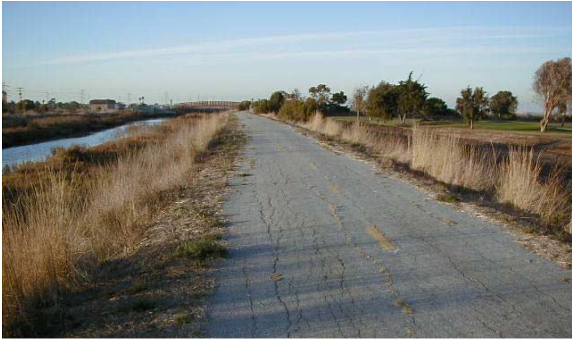
Photo 2-2-- Levee Restoration portion of the project. This photo shows the bike trail that is on top of the Palo Alto side of the levee. This bike trail will be replaced in kind after construction has been completed.
