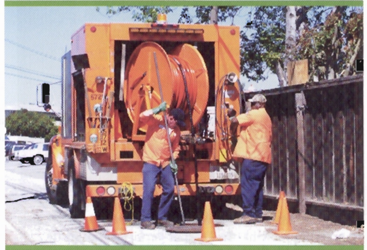
District crew cleaning sewer pipe
