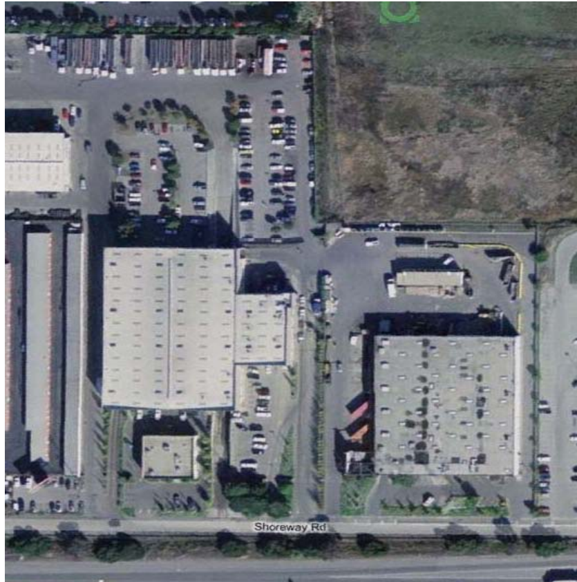
Figure 2-2. SRDC Facility Overview
