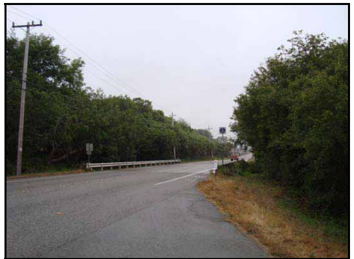
PHOTO 4: Perennial Drainage (Butano Creek) along Pescadero Creek Road, looking northeast.
