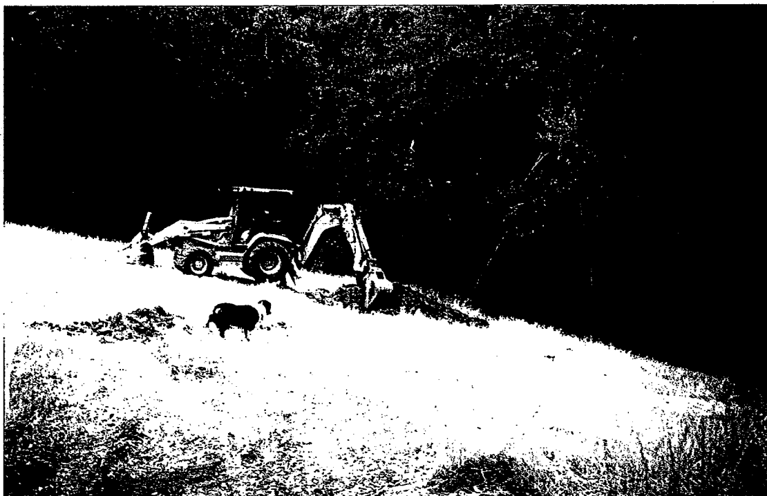
View of northwestern portion of site. Excavating Test Pit 15.
