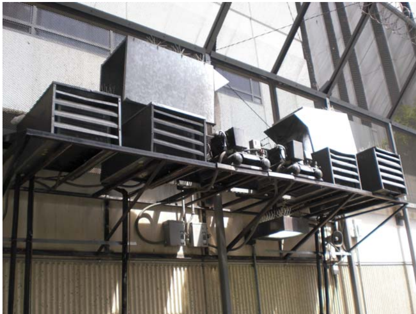
Dock area compressors for kitchen. Refrigerator and freezers are mounted too high for proper maintenance
