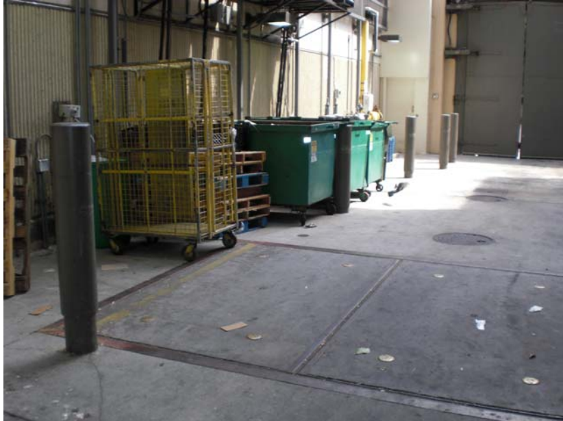
Shared receiving and trash dock is a daily food safety challenge
