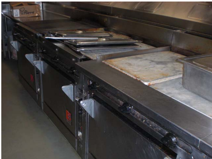
Gas cooking line is at the end of its useful life and needs to be replaced - $45,000
