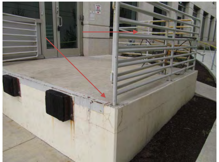
PHOTOGRAPH 20 Minor spalling at the loading dock. Note rusted guardrails.
