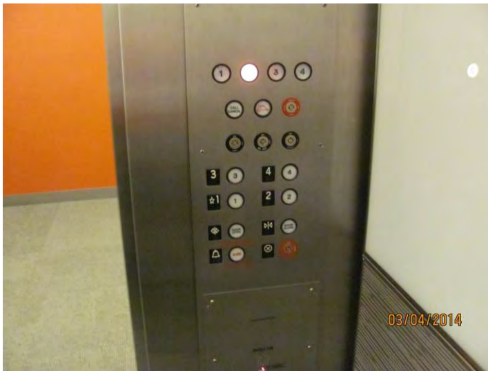
PHOTOGRAPH 85 Car operating panel, ADA Compliant
