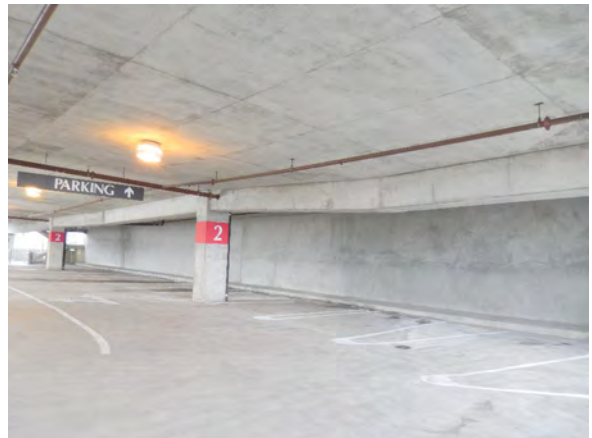
Concrete Shear Walls in Parking Structure
