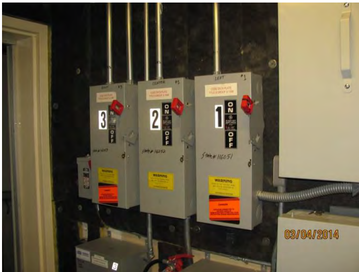
PHOTOGRAPH 101 Mainline disconnect switches, Bldg. II
