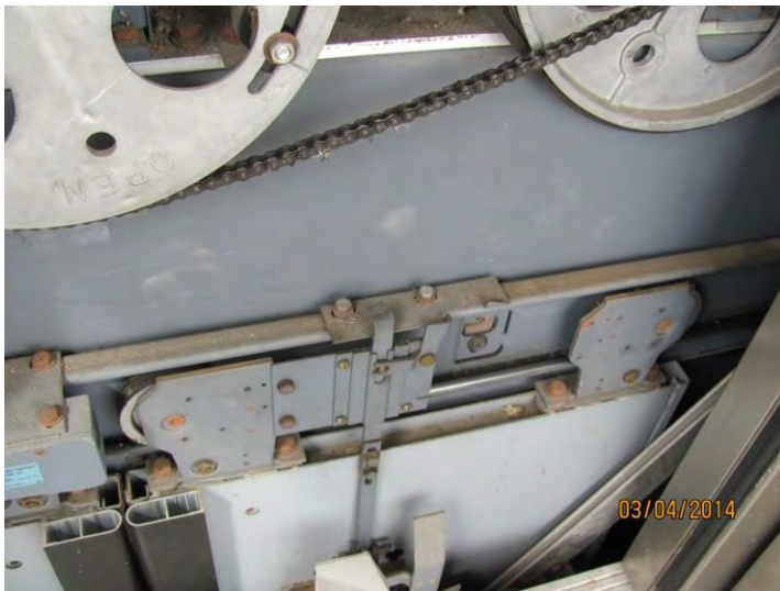
PHOTOGRAPH 97 Door restrictor device, Garage Car
