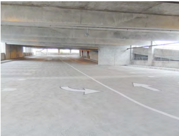
Typical Concrete Beams and Slabs in Parking Structure
