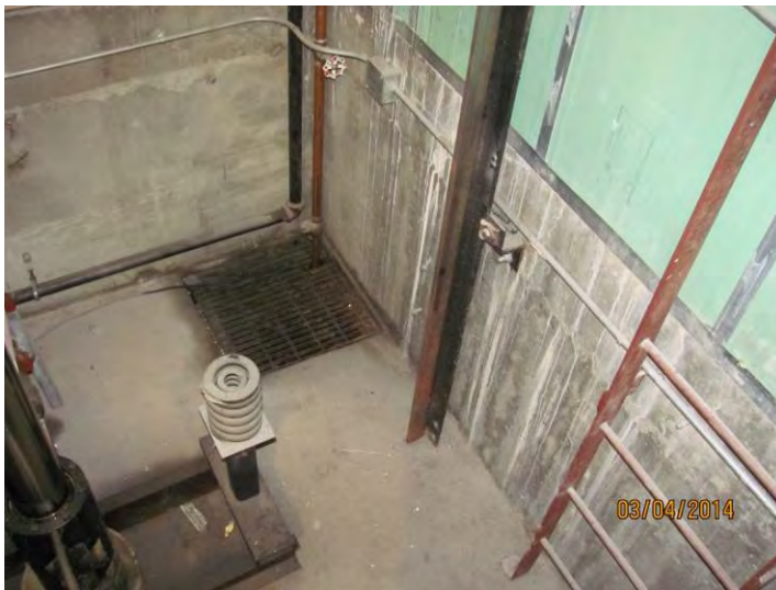
PHOTOGRAPH 87 Proper pit access ladder and sump pump
