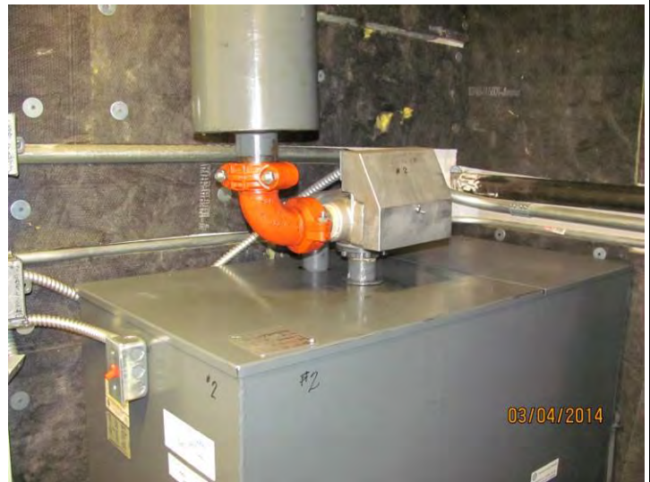
PHOTOGRAPH 102 Typical EECO hydraulic pump unit, Bldg. II
