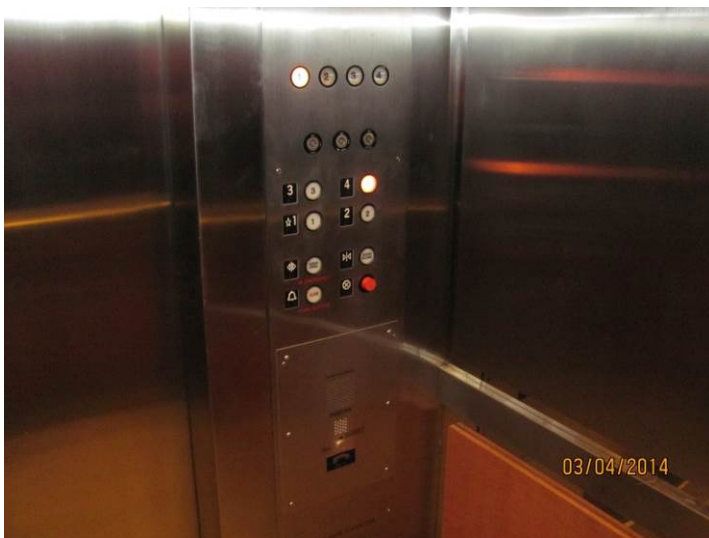
PHOTOGRAPH 103 Car operating panel, Bldg. II
