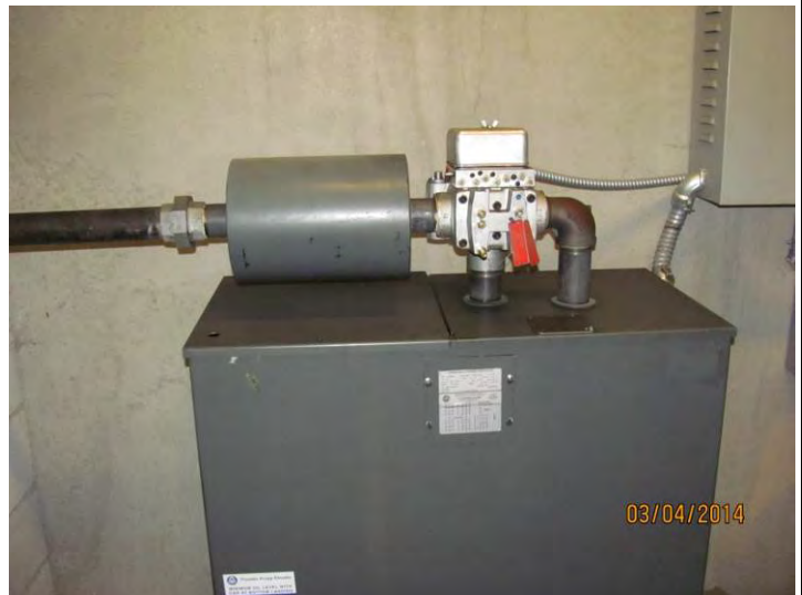
PHOTOGRAPH 100 EECO hydraulic pump unit, Garage Car
