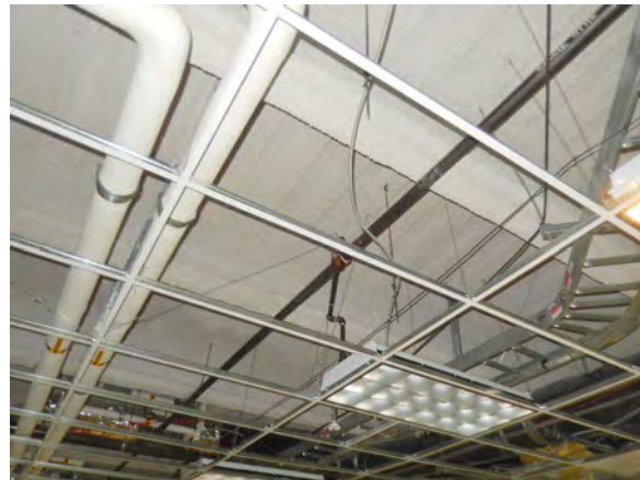
Typical Elevated Floor Framing with Corrugated Metal Deck and Steel Beams
