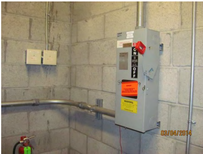
PHOTOGRAPH 99 Mainline disconnect switch, Garage Car
