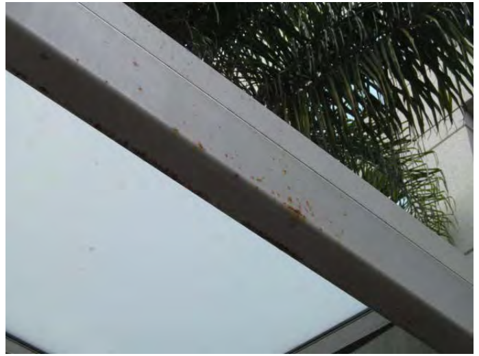
PHOTOGRAPH 18 Minor rust on the metal canopy structure between the two buildings
