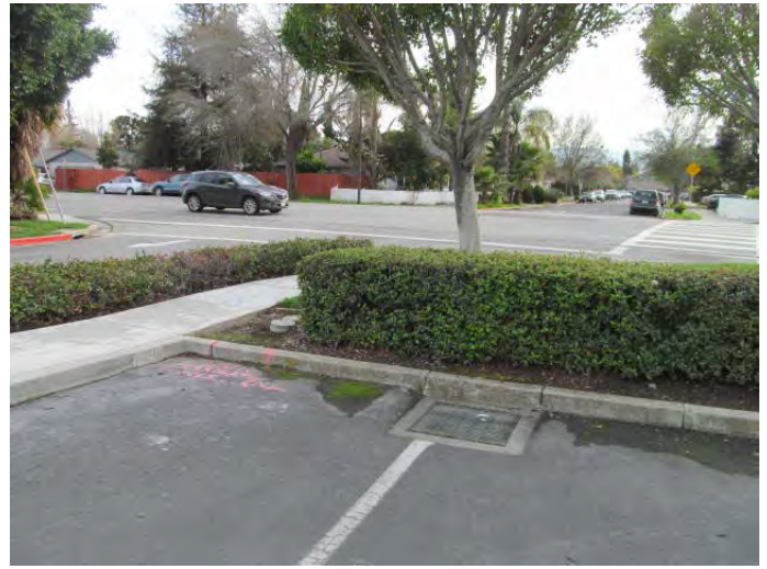
PHOTOGRAPH 10 Catch basins on site for storm water drainage
