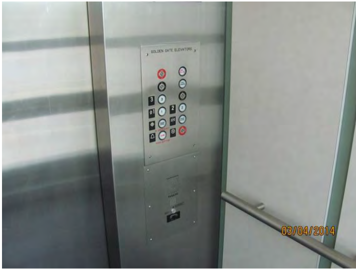
PHOTOGRAPH 93 Garage Car operating panel
