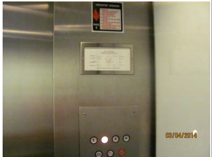
PHOTOGRAPH 86 Car position readout and fire service controls
