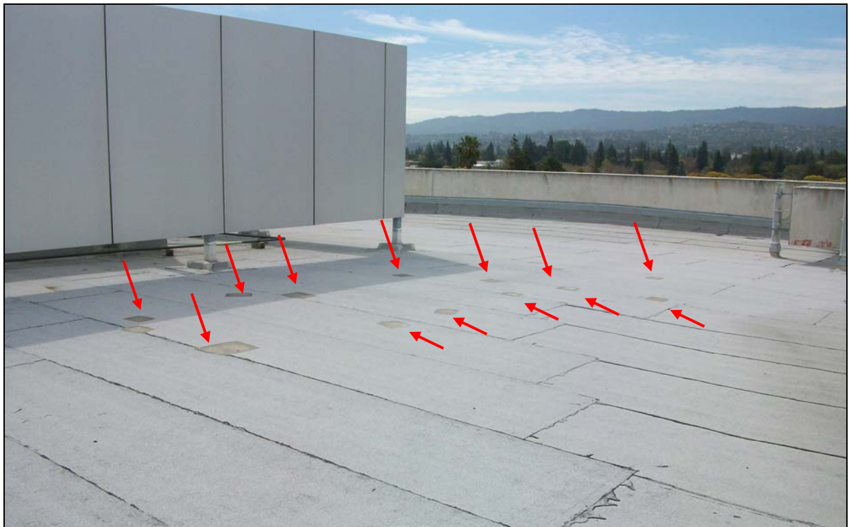
Previous Repairs (Small)
