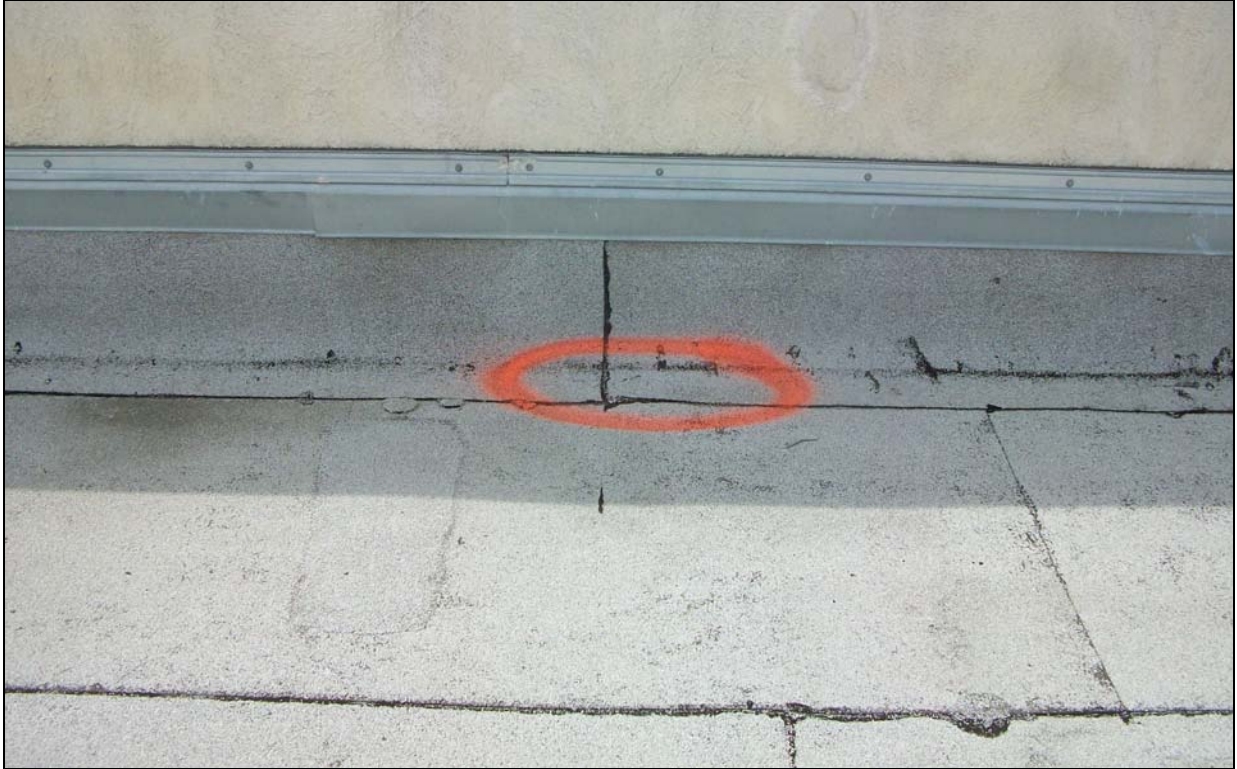
Base Flashing Blisters
