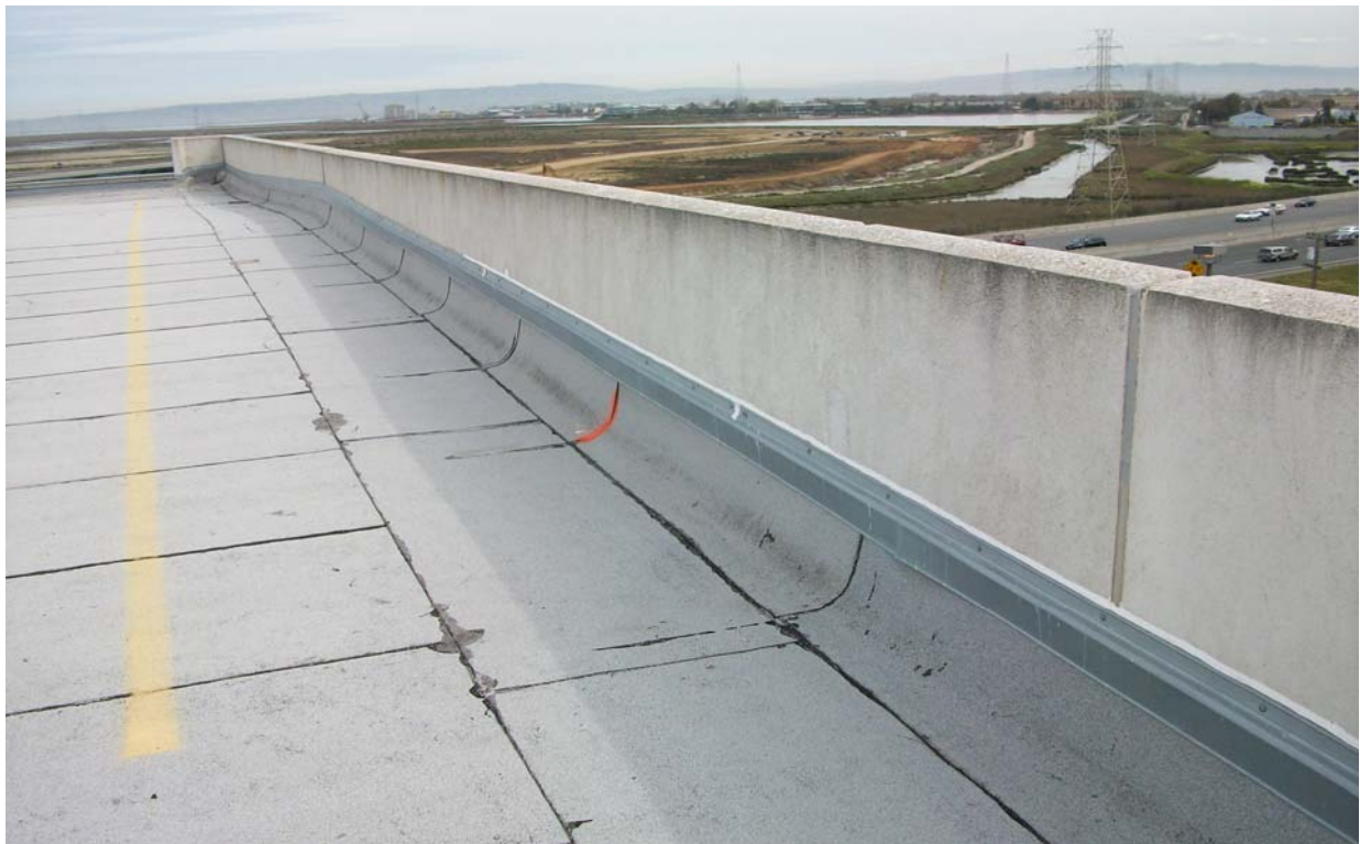
Open Base Flashing Seams
