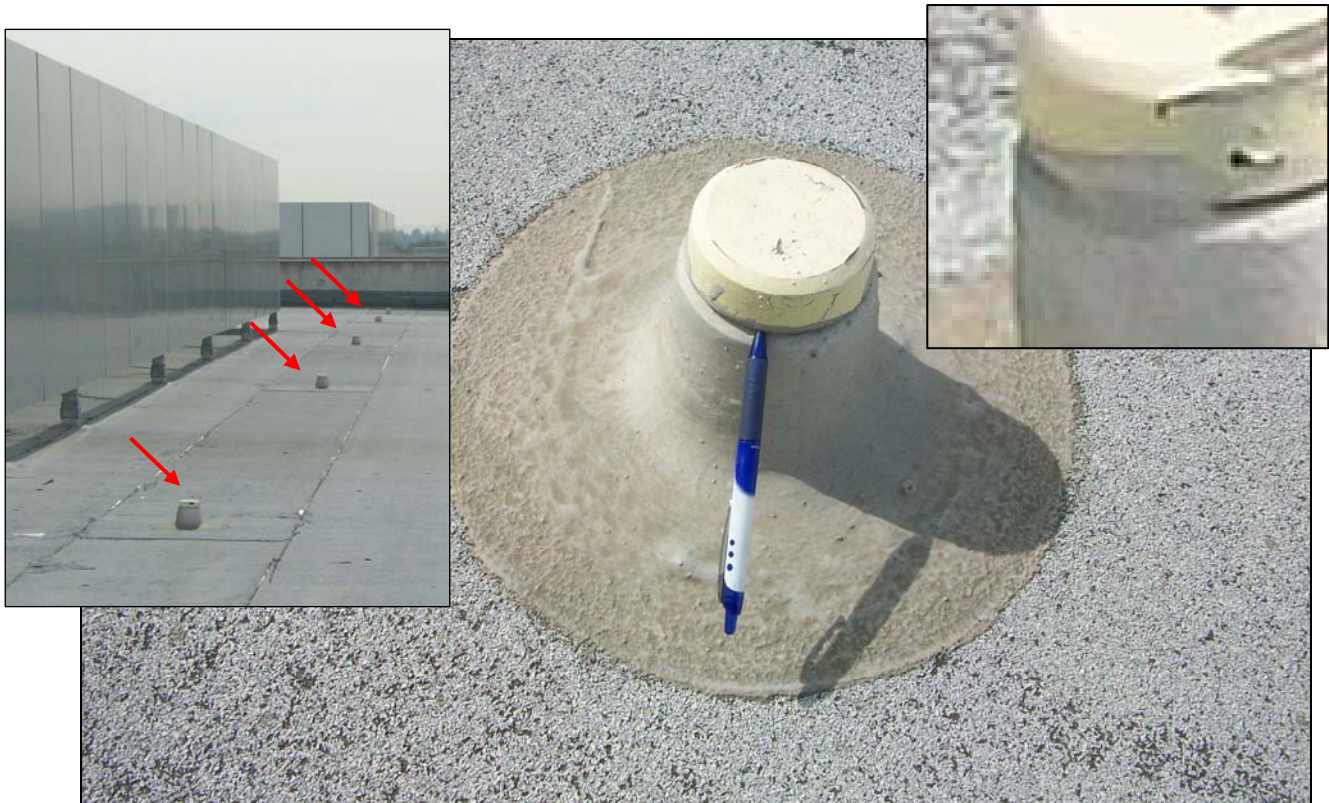
Breather Vent Missing Cap
