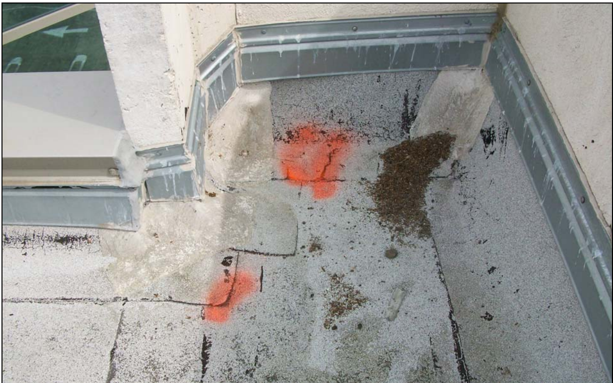
Base Flashing Repairs
