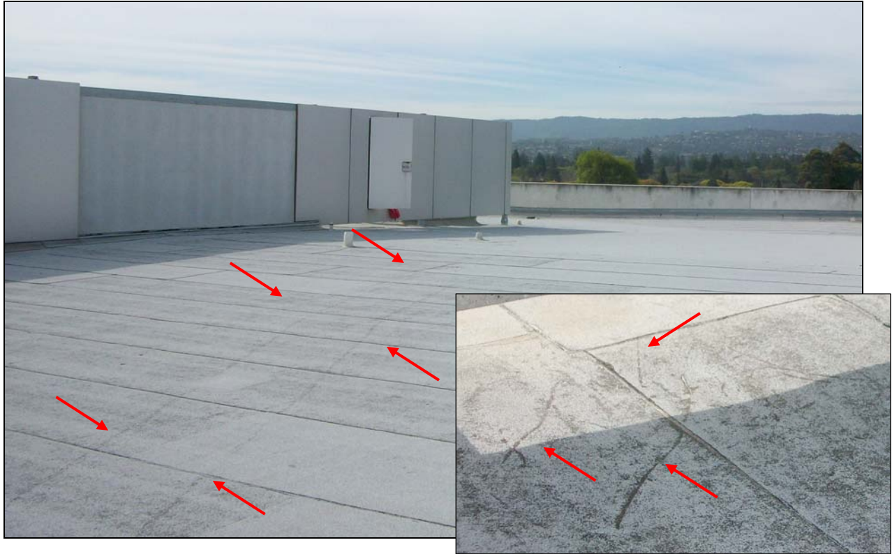
Membrane Scoring (poor care by service personnel)
