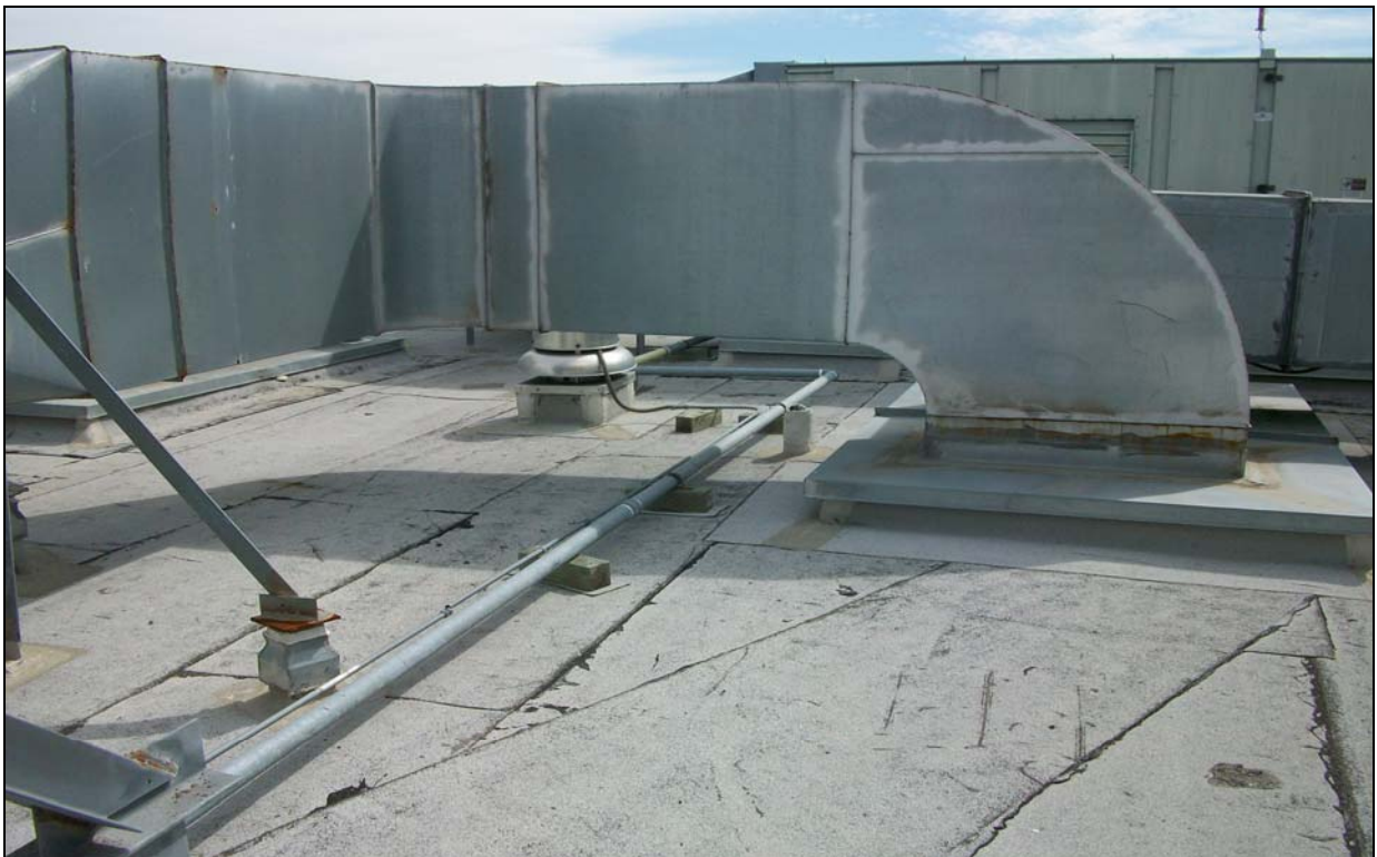
Cap-Sheet Scoring (Mechanical Service Personnel)
