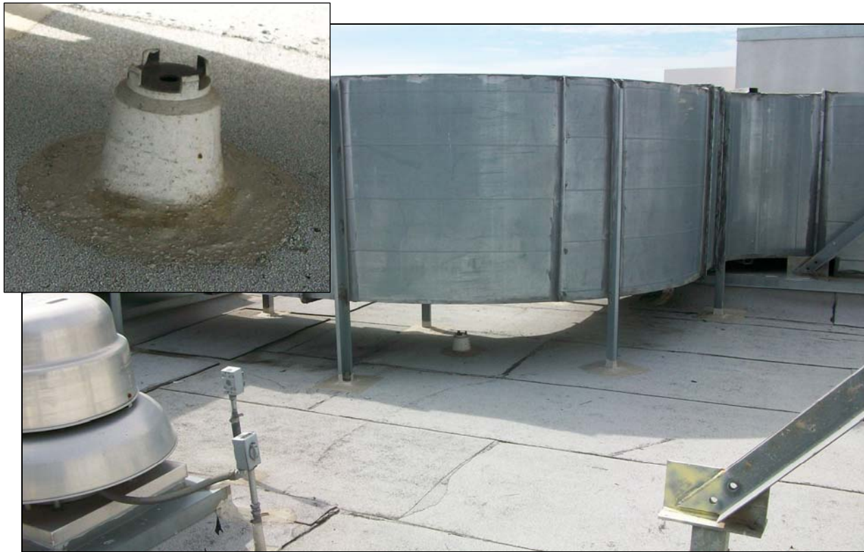
Breather Vent Missing Cap
