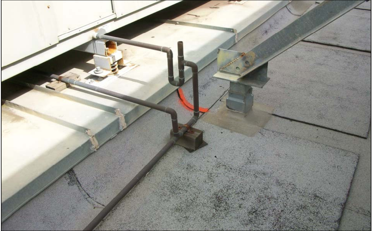
Open / Exposed Base Flashing Seams
