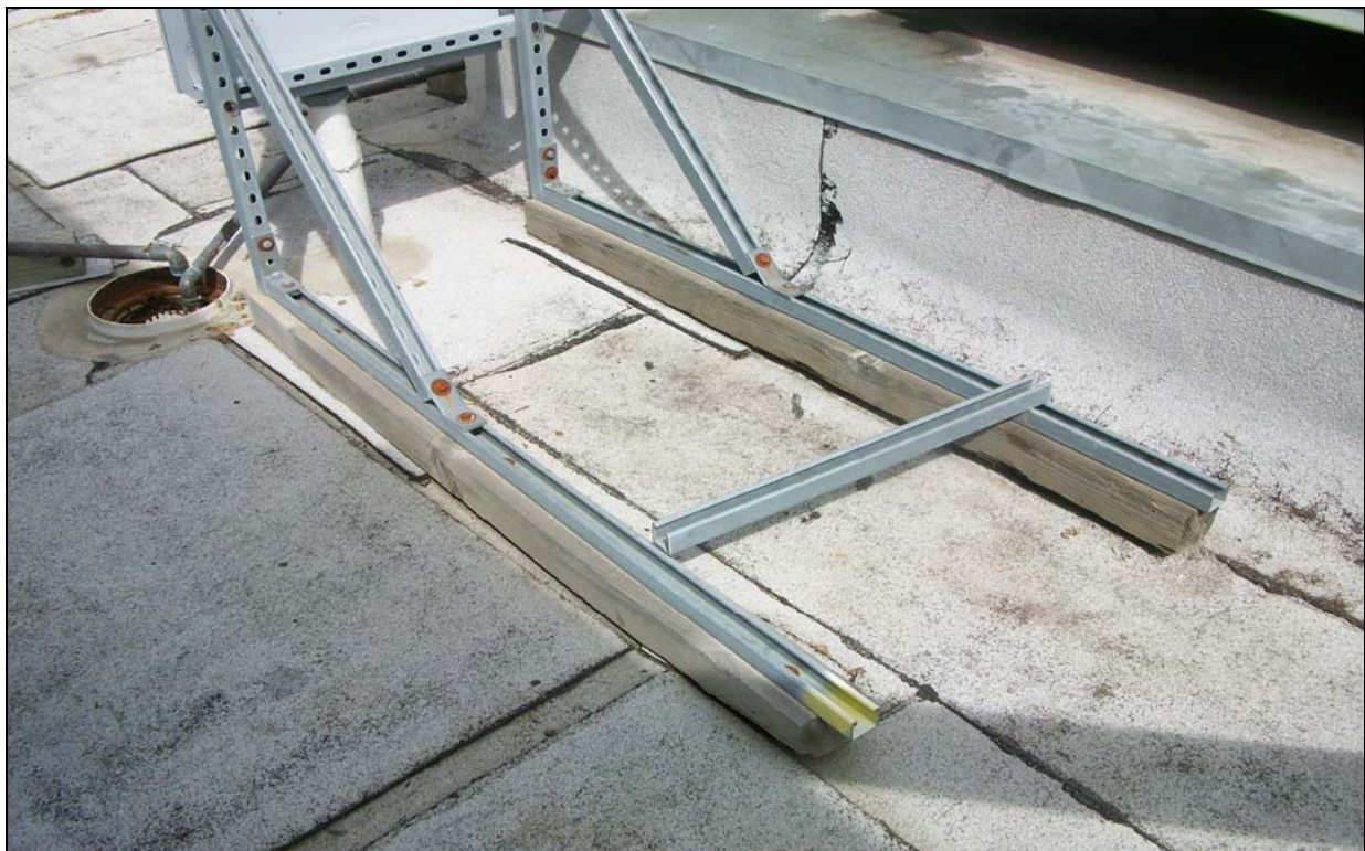
Electrical Box Installations – Unequal Weight Distribution (typical)
