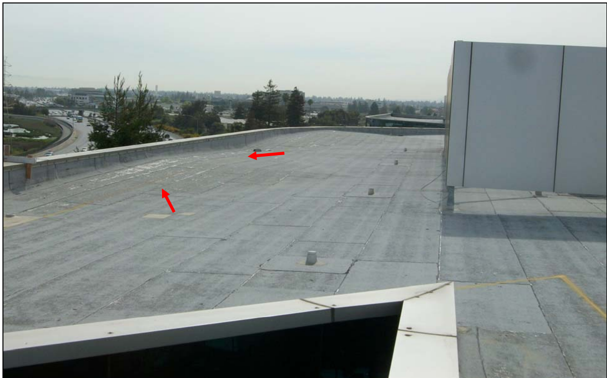
Extensive Granule Loss
