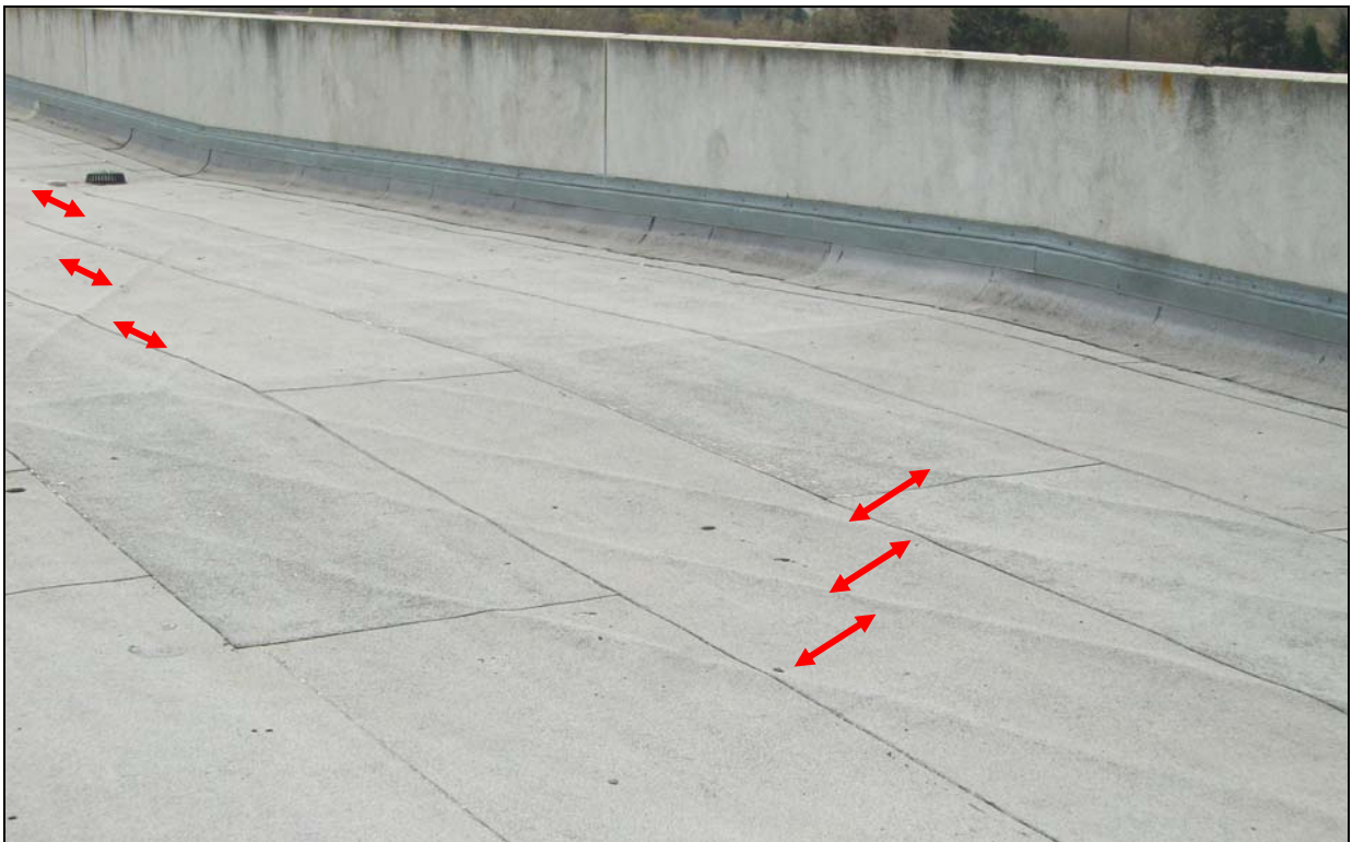
Underlying Membrane Ridging (close-up)
