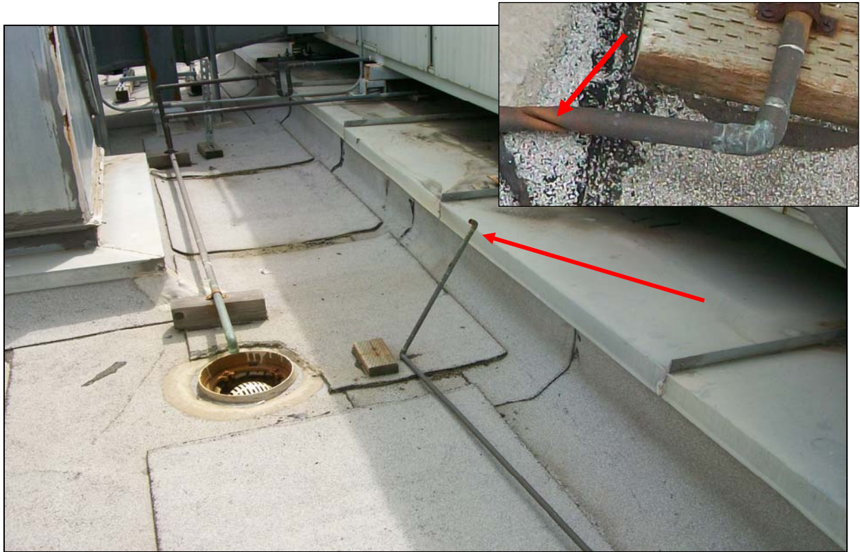
Bent / Obstructed Condensation Line
