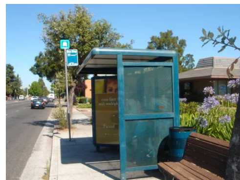
Figure 4-2: Poor Placement of Street Furniture Limits Sidewalk Width
